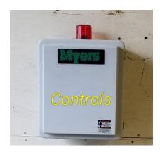
The control panel box to your grinder pump is located on the side of your home that measures approximately 12" and has a red alarm light on top. This box must be visible at all times and easily accessible, as service and maintenance will also be done through access to this box. If you observe the red light on at any time, it indicates a problem. Notify the Village immediately and a Village Representative will call you and access the situation.
